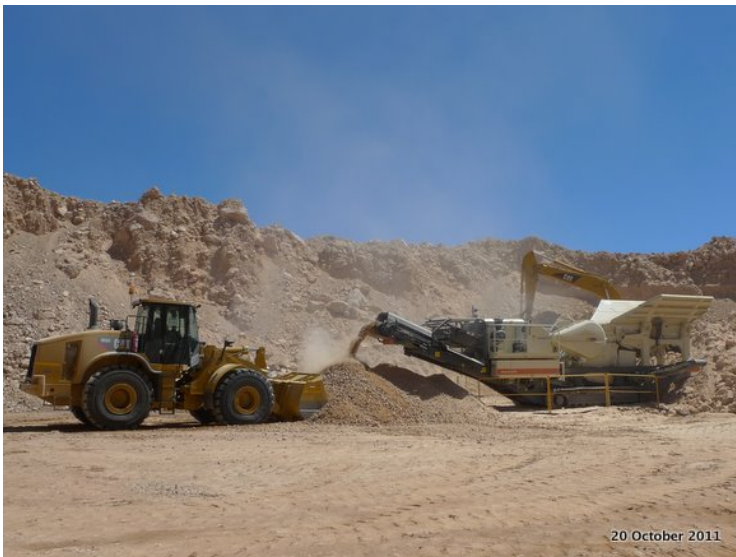
Tshipi Borwa – Waste rock crushing
