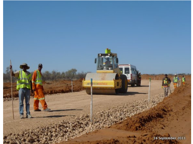
Tshipi Borwa –Railroad siding foundation construction
