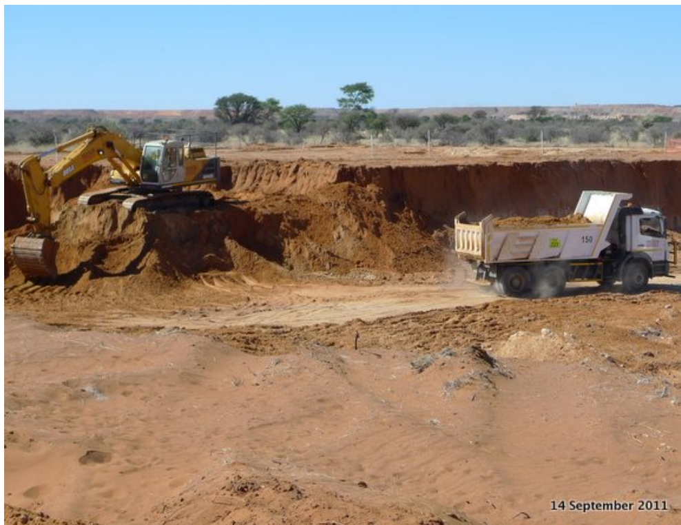
Tshipi Borwa – Storm water pit excavations
